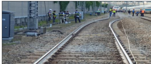
SRT Derailment Accident('22.7)
