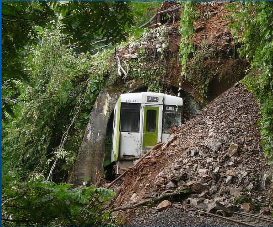
2010 Train derailment due to a landslide on the Iwaizumi Line. Discontinued in 2014
