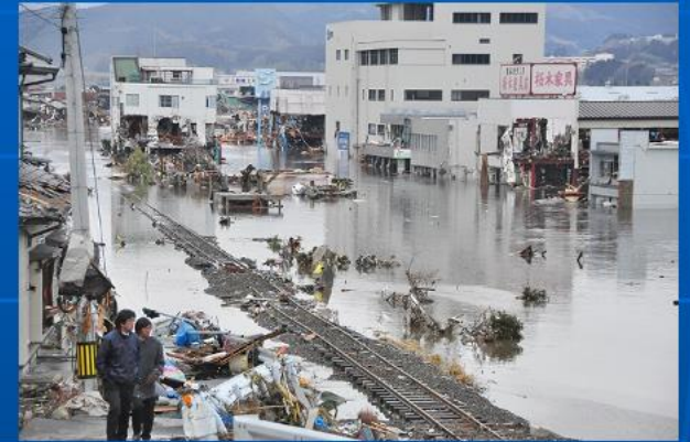
Tsunami damaged along Oofunato line
