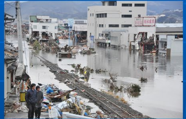
Tsunami damaged along Oofunato line
