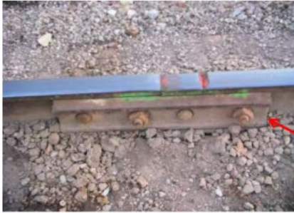
Fish plates / Joint bar
