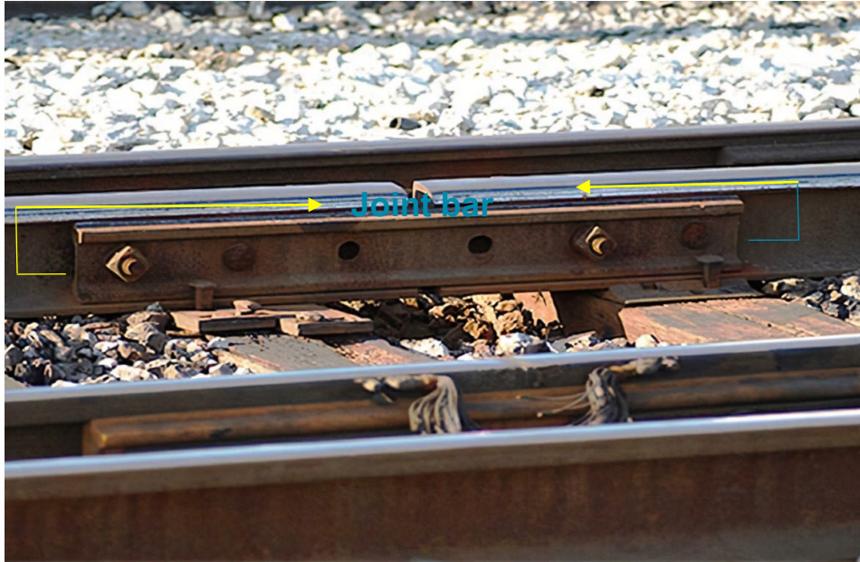
Joint Bar with two Missing Bolts Captured by the System
