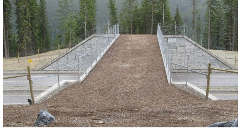
Wildlife overpasses, British Columbia, common for roads than rails. (Photo by B.C. Ministry of Transport, CC BY-NC-ND 2.0)
