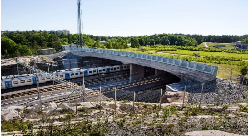
Landscape bridge, in Kallhäll Stockholm (opened 2017), providing a corridor for wildlife to safely pass over the railway. Credit: Mikael Ullén/Trafikverket
