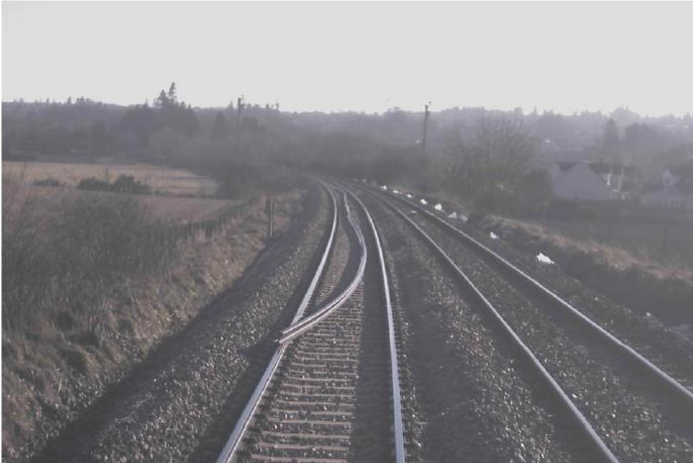
Image from Forward Facing CCTV of train 1E17 showing the rail just prior to impact (image courtesy Virgin Trains East Coast)
