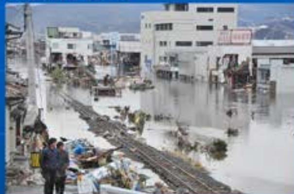
Tsunami damaged along Oofunato line
