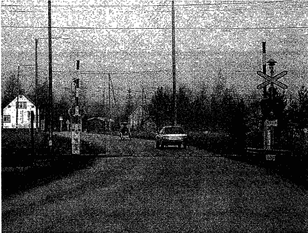
Figure 1. Railway level crossing with half-barriers.
