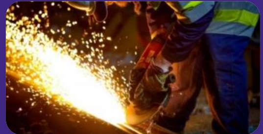
Execution maintenance works
