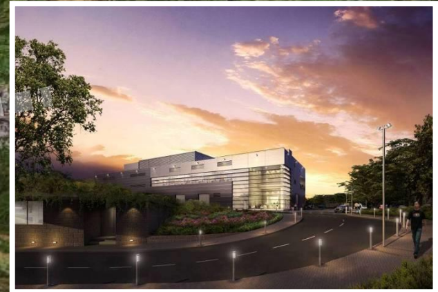
Shek Kong Stabling Sidings & Emergency Rescue Station
