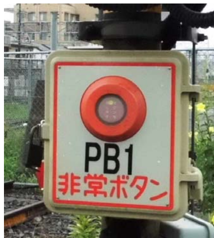
Photo 5: Appearance of level crossing warning systems (Emergency push button)
