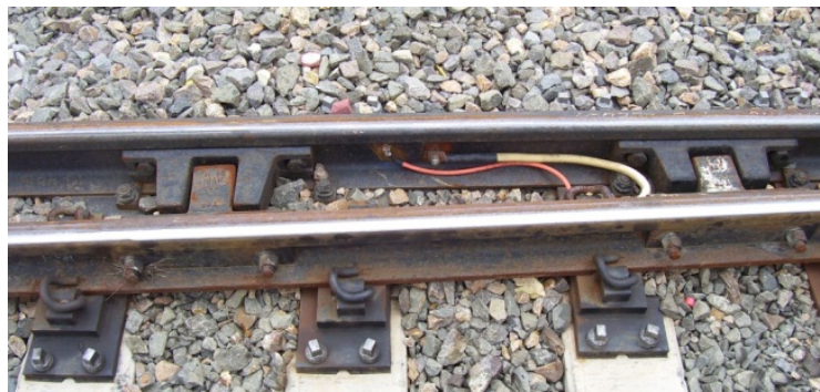
Figure 6: The VAE turnout's double anti-creep device
