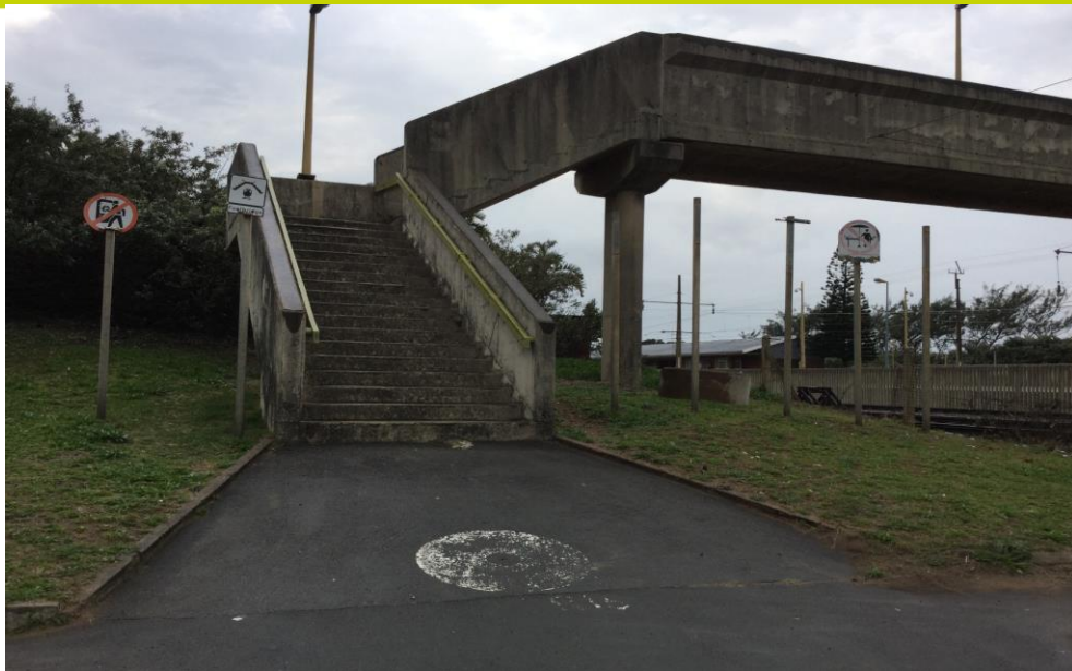
Footbridge at a Station
