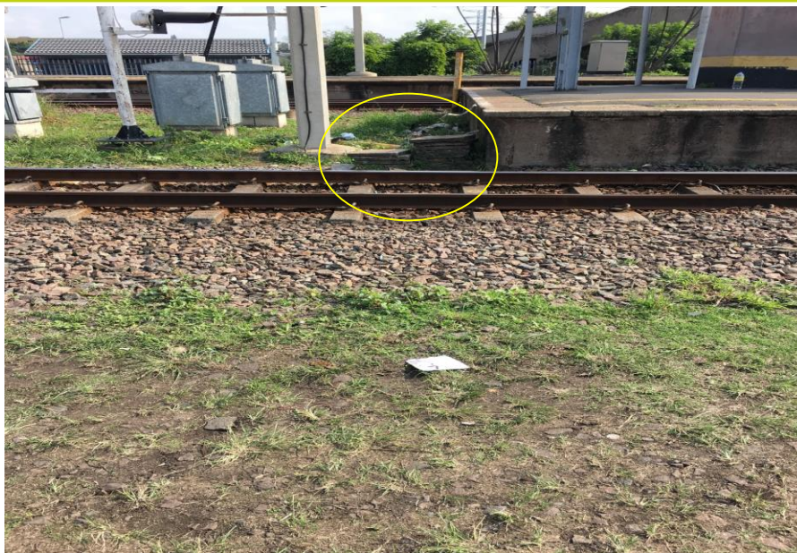
Steps added to gain access to the platform
