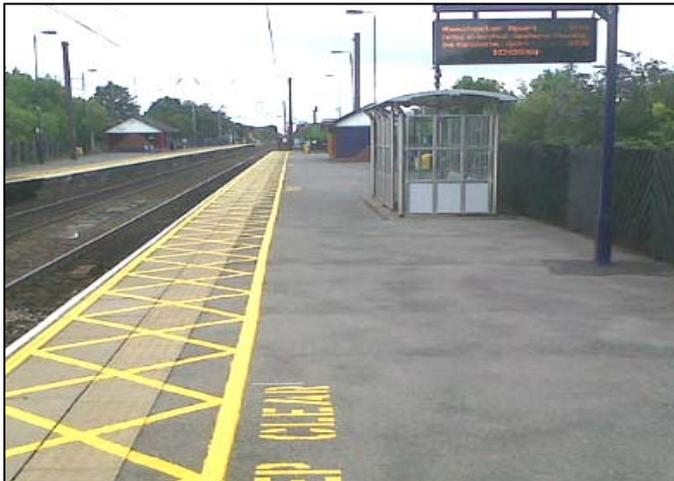
**Figure 5: Platform edge hatching at Northallerton station**
