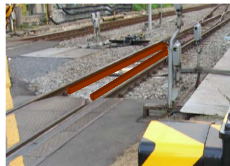
Image 4: Guard for prevents deviation (An example of countermeasure against secondary damage from level crossing accidents) Note: We will test and analyze the effect of these ideas on the experimental line.
