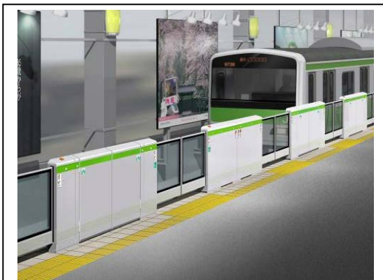
Image 3: Platform edge doors
