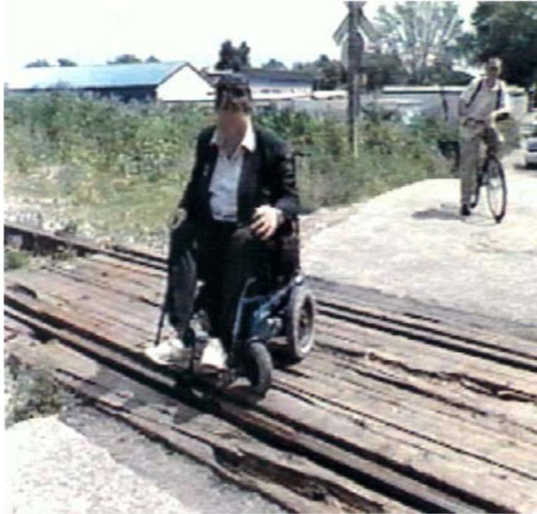
**Photo 3 (Perishable Data) Image taken from a Media Videotape of Deteriorated Crossing Planking**
