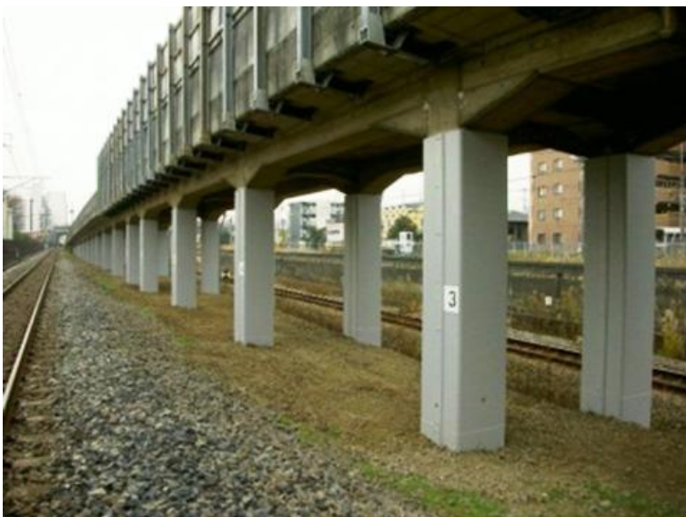
Figure 9: Reinforced Elevated Bridge against Severe Earthquake
