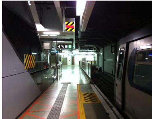
Figure 9: Vertical stopping mark at Hung Hom Station
