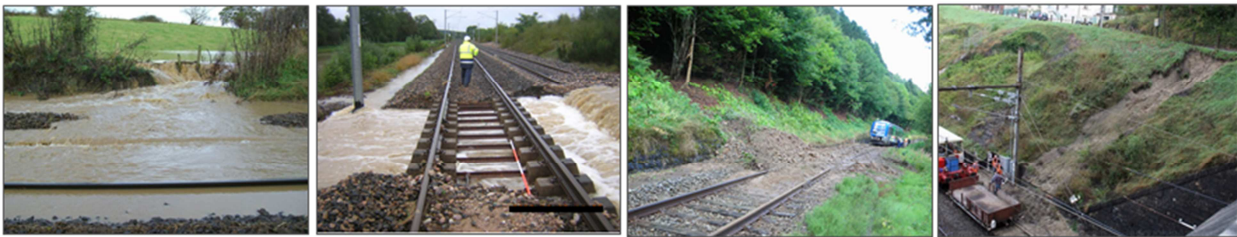
Figure 1: Photos of incidents on railways caused by surface runoff. From left to right: flood, ballast transport, mudslide and slope failure.
