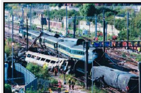
Ladbroke Grove (UK) Slanting collision - 1999
