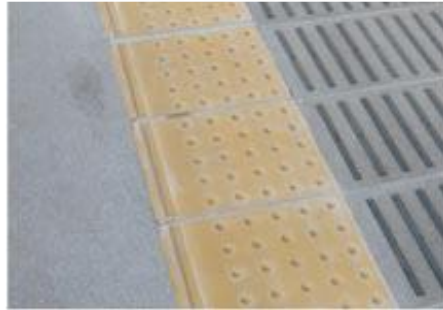
Figure 7: Braille blocks with embossed lines indicating the inward side of the platform
