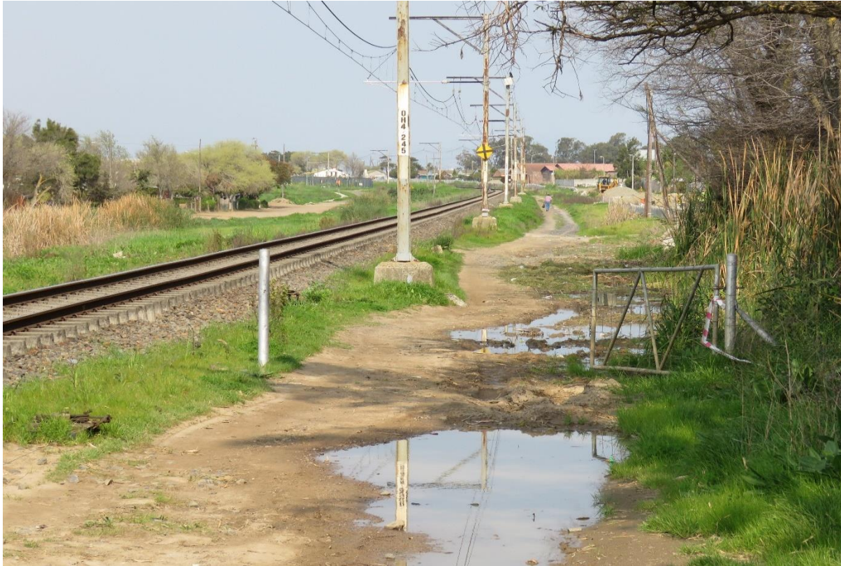
Figure 4: The sight distance to approaching trains from the road stop line is excellent
