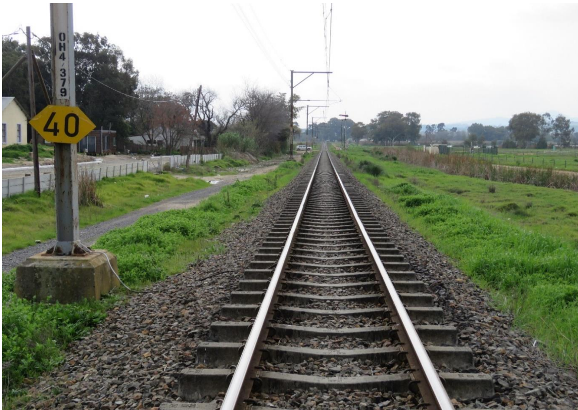
Figure 2: This is the view that the train driver would have had of the crossing from the second whistle board (125m). A vehicle, which has stopped at the crossing, can be seen in the distance The 40km/h speed board was erected after the accident on the instruction of the RSR
